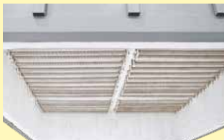
Heating elements in furnace hood
