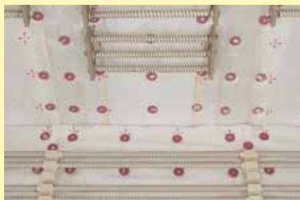
Fabric cover on the fiber roof (and sides) to reduce fiber dust
